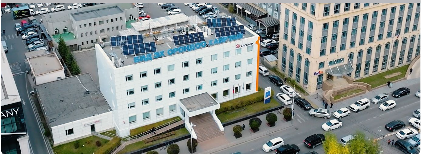
Solar installation at XacBank central offices, Ulaanbaatar, Mongolia.
