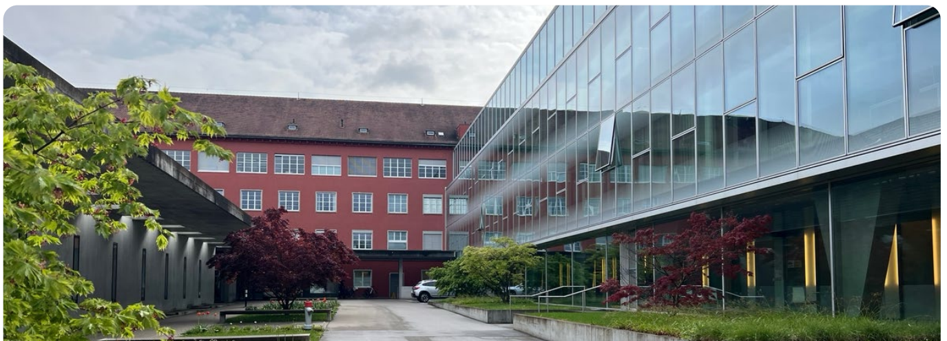
The Stiftung Diakoniewerk Neumünster, which includes the Zollikerberg Hospital (Spital Zollikerberg), is working hand in hand with the Servetia team, exploring options towards decarbonisation through as-a-Service models, from heating and cooling to lighting systems and photovoltaic solutions.
