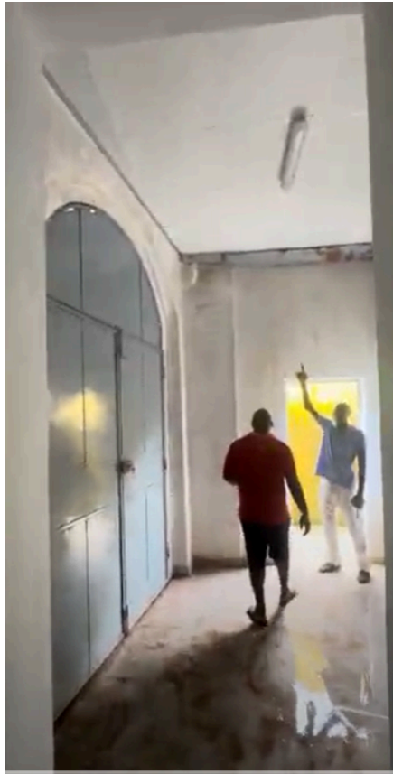
“Recepcao” room. One of the two rooms available for being transformed into a cooling chamber
