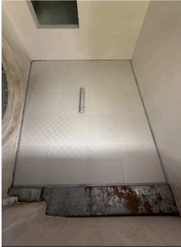
Ceiling details of "Recepcao" room
