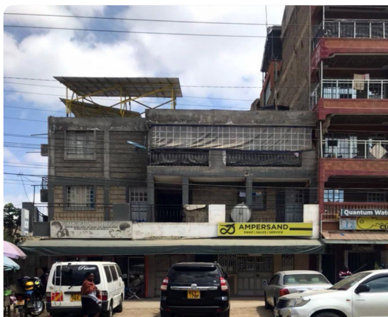
Street view of the pilot (Panels top left). Source: Ampersand
